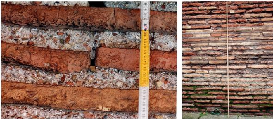
From left to right: Detail of the wall face on the south-west side of the Basilica di San Vitale, Ravenna; external wall face of the Basilica di San Vitale where restoration works are visible. Photos by Nora Lombardini, from PhD Thesis by Nora Lombardini.
