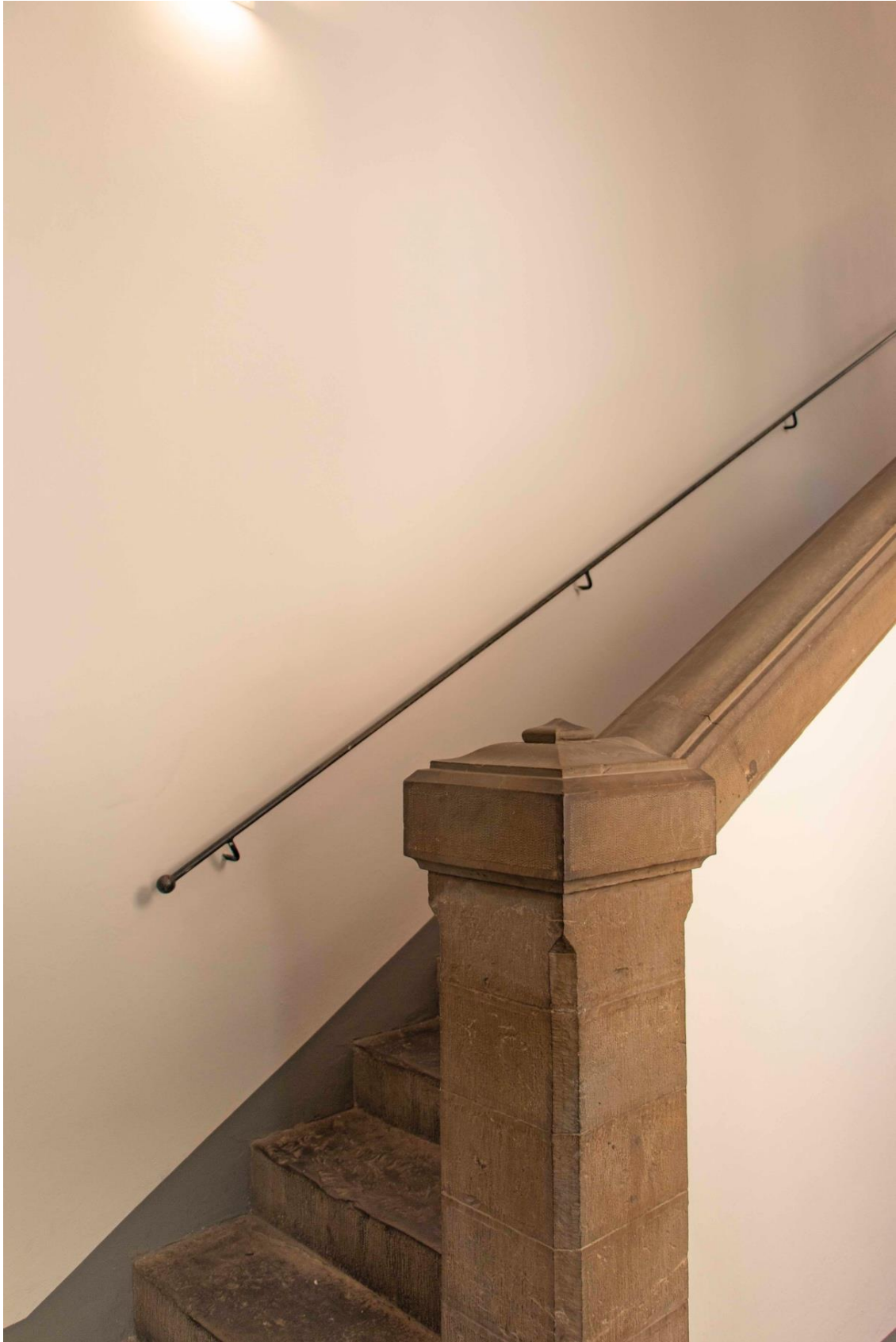
Figure 10: Detail of the staircase distributing the museum's floors, finished in the traditional pietra serena. Photograph by Corinna del Bianco.
