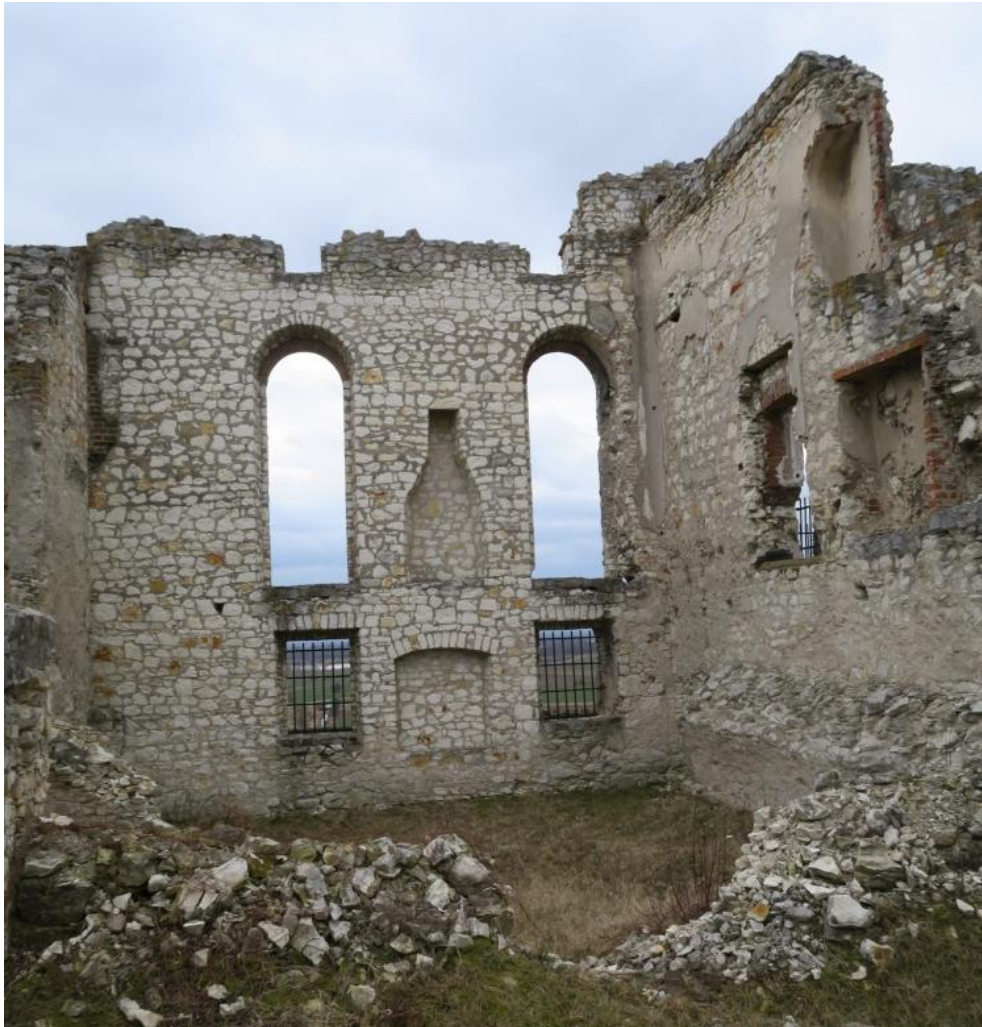
Destruction of the historical substance. Photo by A. Fortuna-Marek
