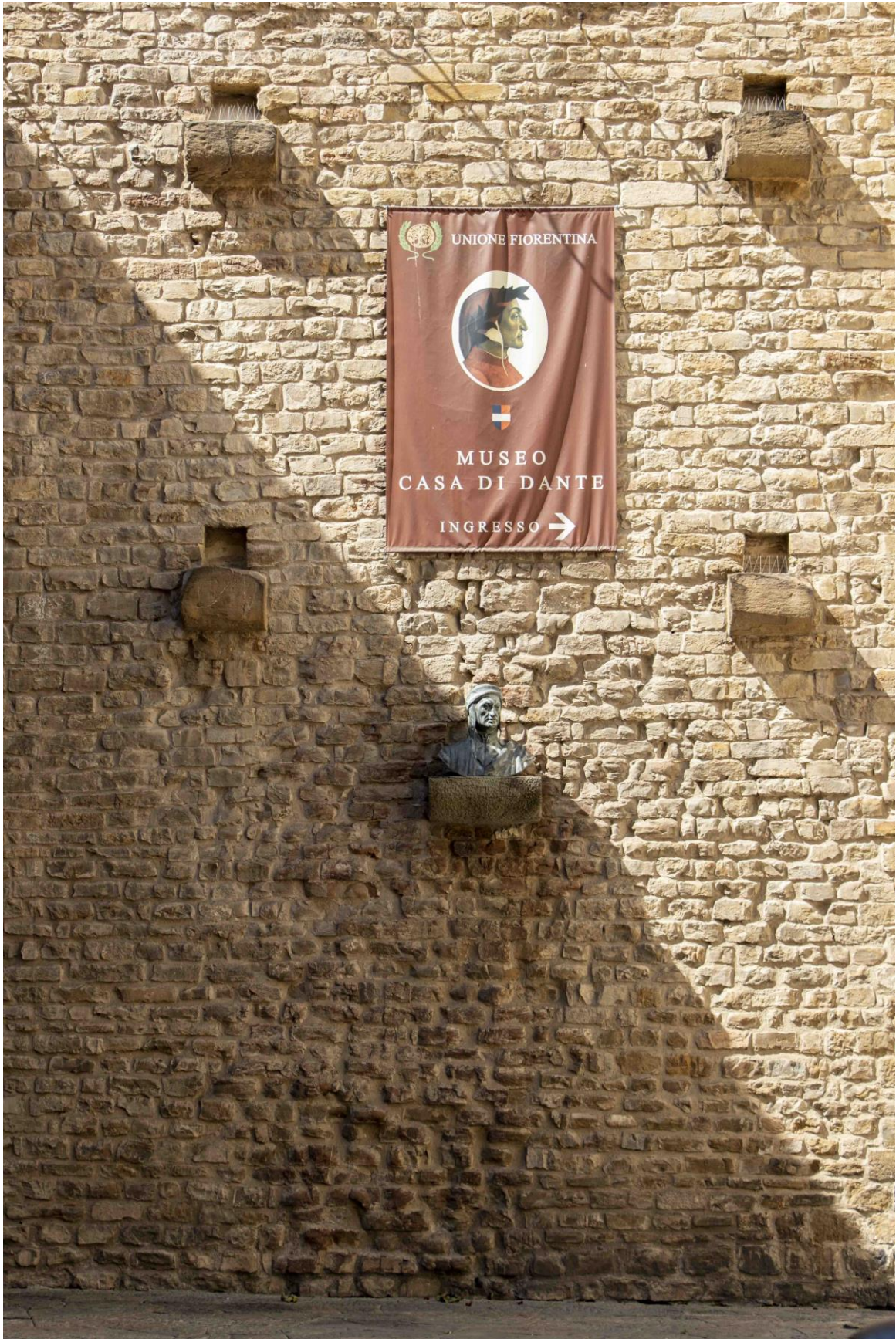
Figure 2: View of the façade of the tower covered in pietraforte , with putlock holes, Dante's bronze bust and the indication for the entrance located on the side of the tower. Photograph taken in the little square in Via Santa Margherita. Photographs by Corinna Del Bianco.
