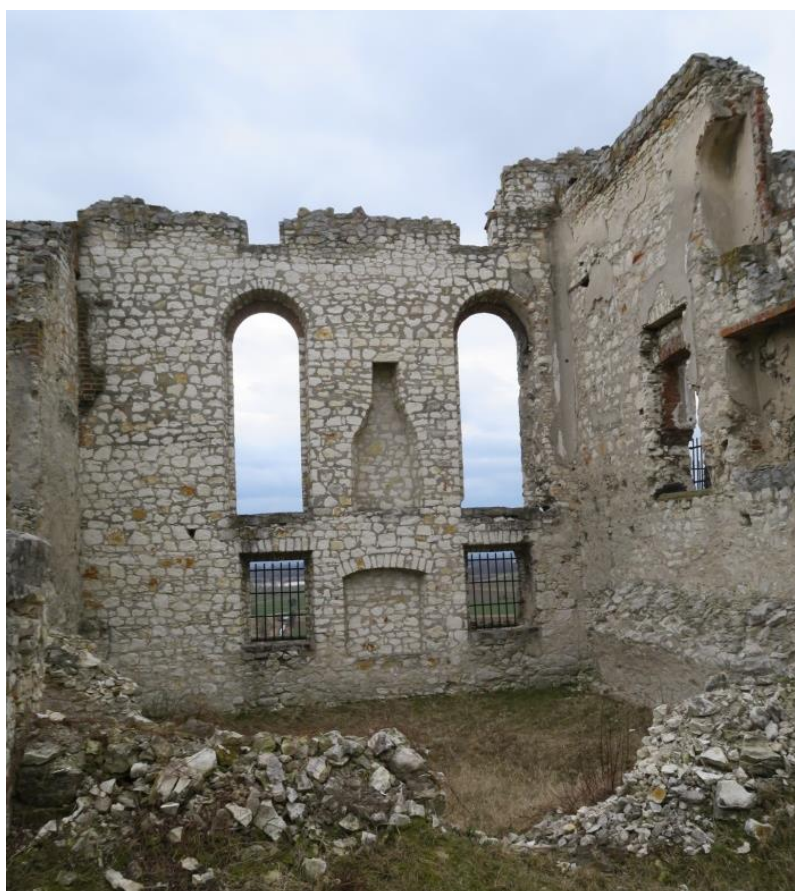
Destruction of the historical substance. Photo by A. Fortuna-Marek
