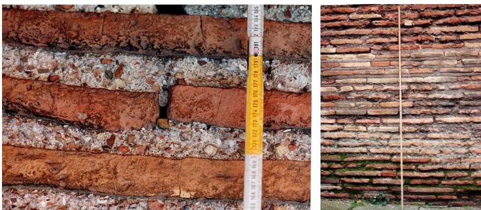
From left to right: Detail of the wall face on the south-west side of the Basilica di San Vitale, Ravenna; external wall face of the Basilica di San Vitale where restoration works are visible. Photos by Nora Lombardini, from PhD Thesis by Nora Lombardini.
