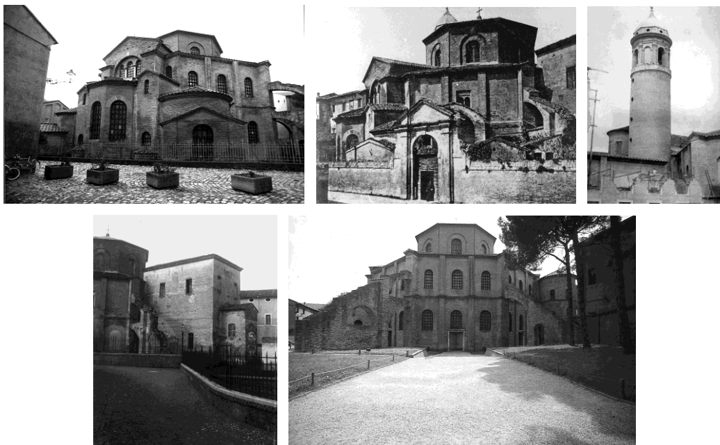
The chapels and the pharmacy built around St Vitale and their demolition during the philological and historical restoration by C. Ricci (pictures from the Archive of Soprintendenza at Ravenna). First and last pictures: views of the Basilica (pictures by Nora Lombardini).
