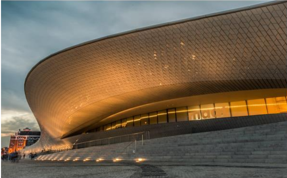
Figure 12 - Sunset and night lighting on the south facade (net 10)
