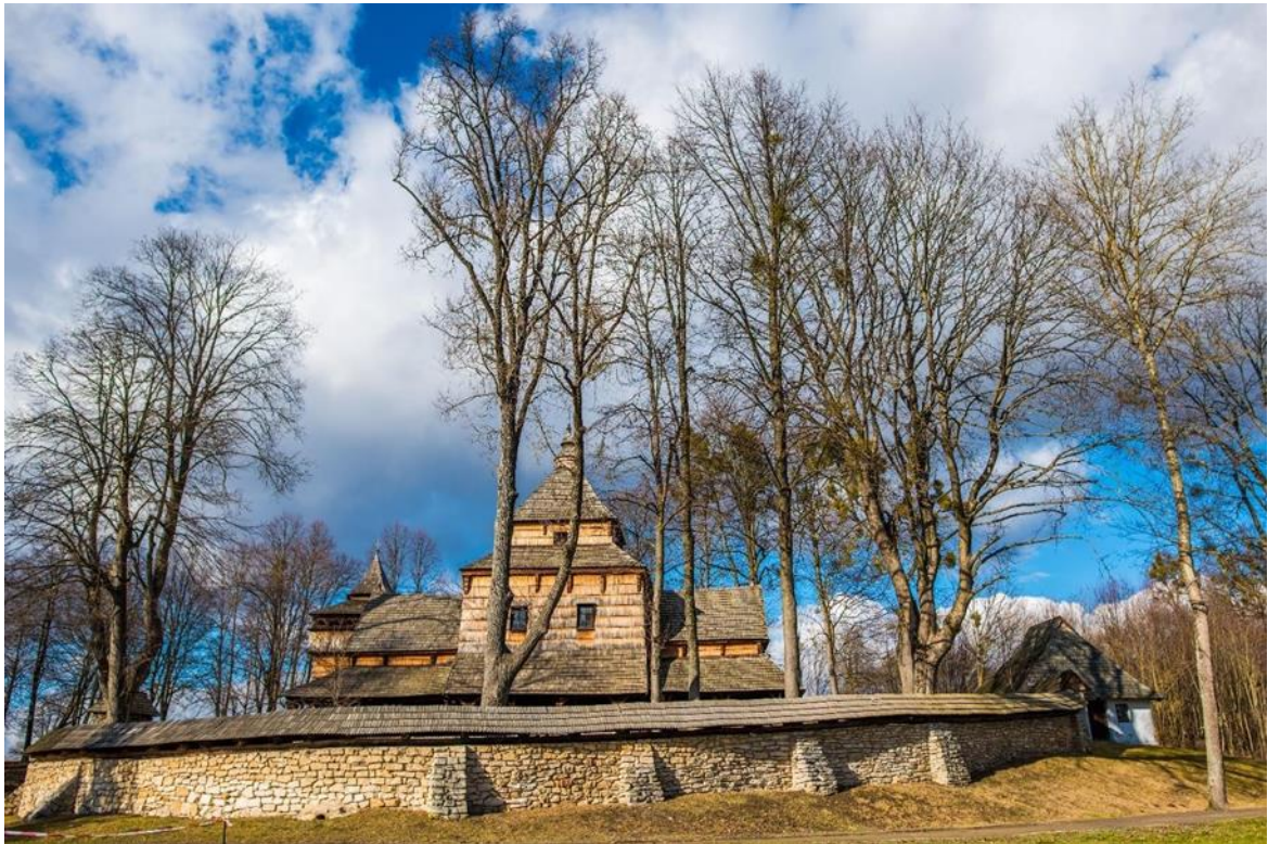
Fragment of the stone fence of the Orthodox church complex in Radruż (from the eastern side). photo. Alicja Mróz, 2020
